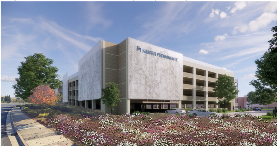
Figure 8: Northeast side of the Parking Garage (Facing Lead Hill Bl./Eureka Rd.)
