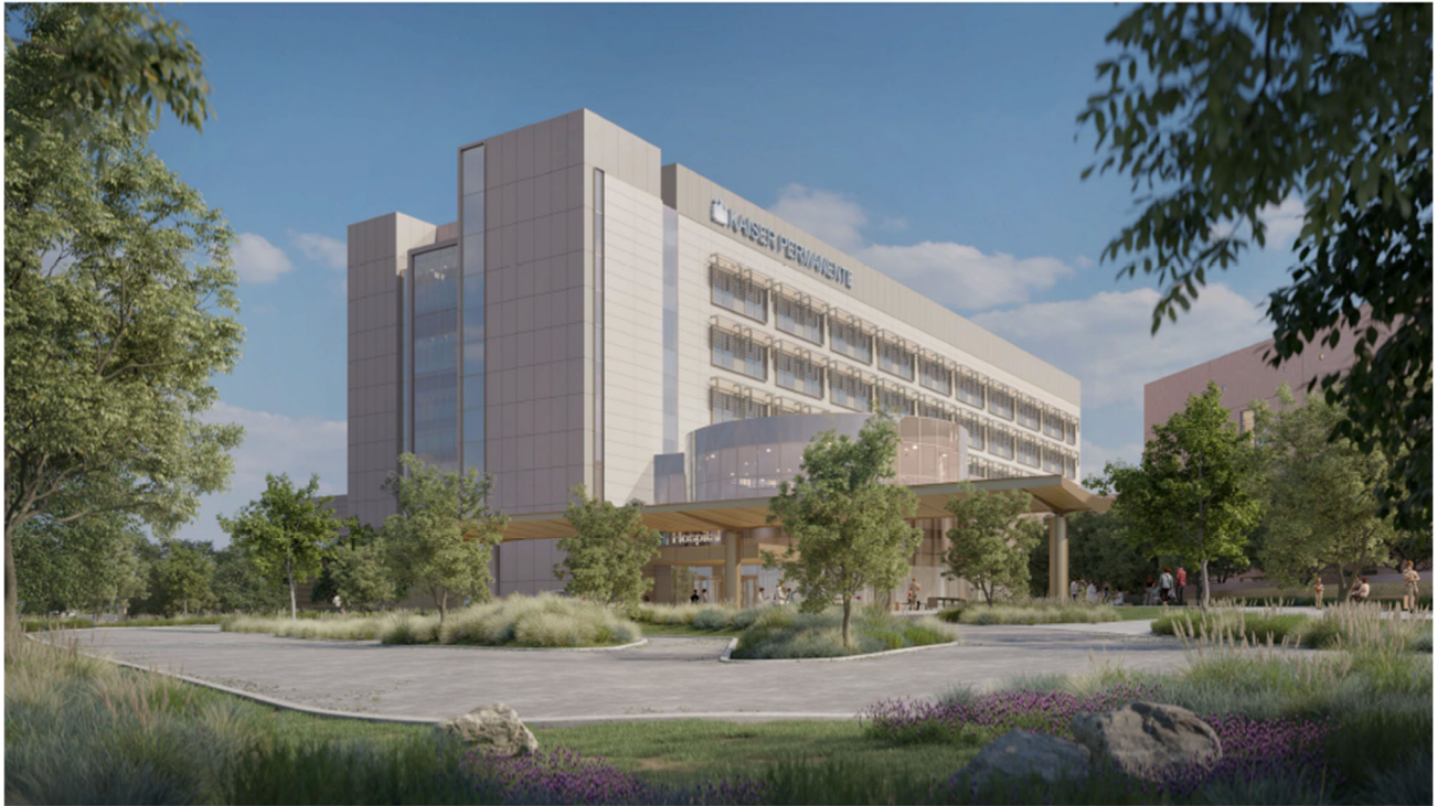
Figure 6: Southwest side of the Inpatient Bed Tower near Hospital Entry
